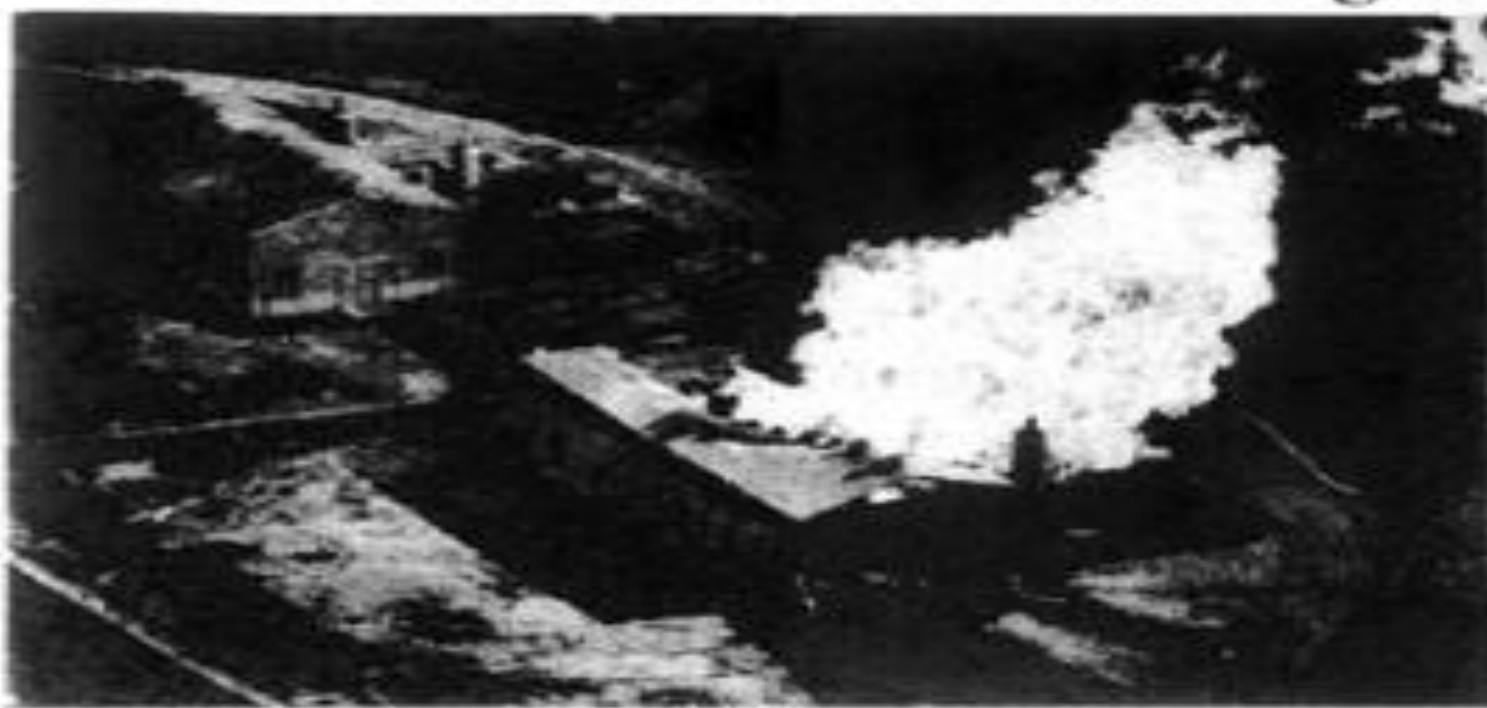
Aerial view of Exxon's compressor station only minutes before gas was shut off
